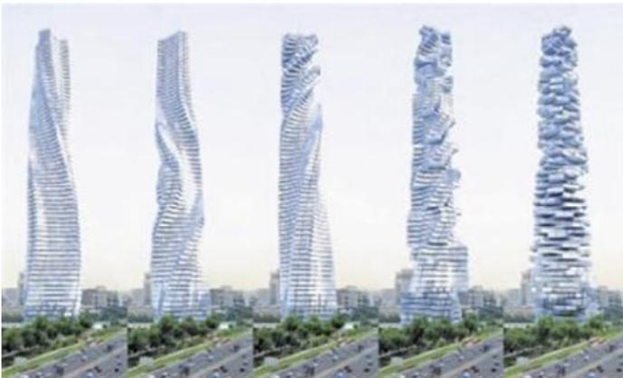
Environment Friendly building. The 420-metre (1,378-foot) building's apartments would spin a full 360 degrees, at voice command, around a central column by means of 79 giant power-generating wind turbines located between each storey.
